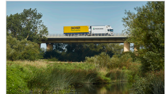
Frigoscandia specialises in temperature-controlled transport and warehousing, with 75 years of experience when it comes to food logistics for fresh, chilled and frozen food, deeply rooted in sustainability. We are the market leader in temperature-controlled food logistics in the Nordics and work to integrate sustainability principles into all dimensions of our operations.
